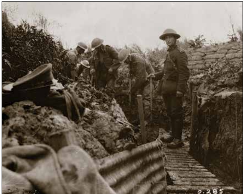
Repairing trenches, 22nd Infantry Battalion, July 1916.
